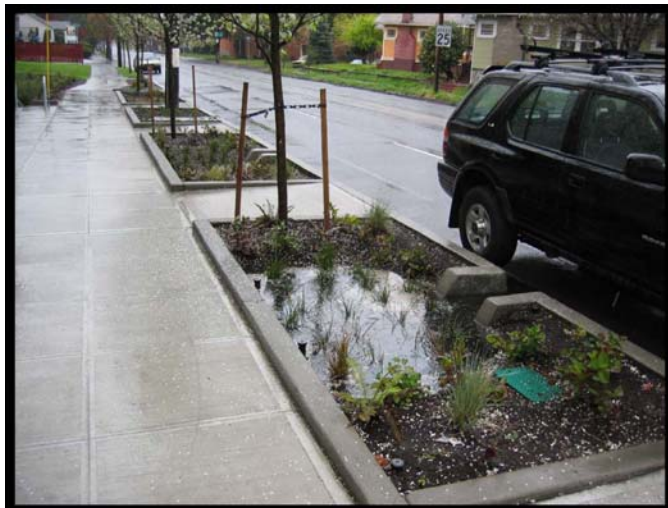
Figure 4. Bioretention areas along a street in Seattle (image provided by Greenworks)
