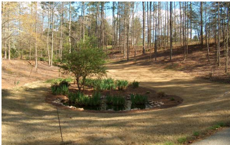
Figure 2. Typical bioretention area appearance (Photo by R.A. Vick)
