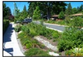
of the strip or swale and is filtered by soil along the way. Incorporate an overflow pipe into the design if necessary.
